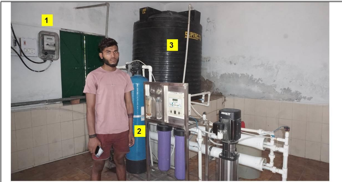
1. Energy Meter. 2. R.O. Plant. 3. Processed Water Storage Tank (2KL).
