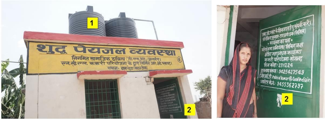
1. Overhead Tank. 2. Contact No. for Complaint & Operator Mobile No.
