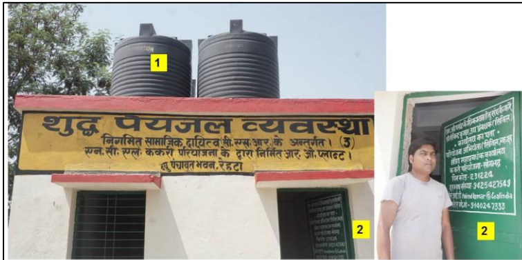
1. Overhead Tank. 2. Contact No. for Complaint & Operator Mobile No. .
