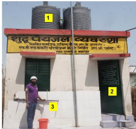
1. Overhead Tank. 2. Contact No. for Complaint & Operator Mobile No. 3. Outlet of Purified Water
