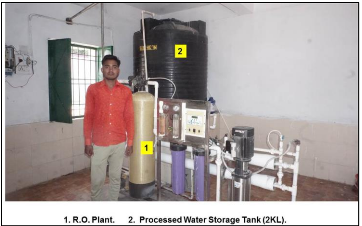
1. R.O. Plant. 2. Processed Water Storage Tank (2KL).
