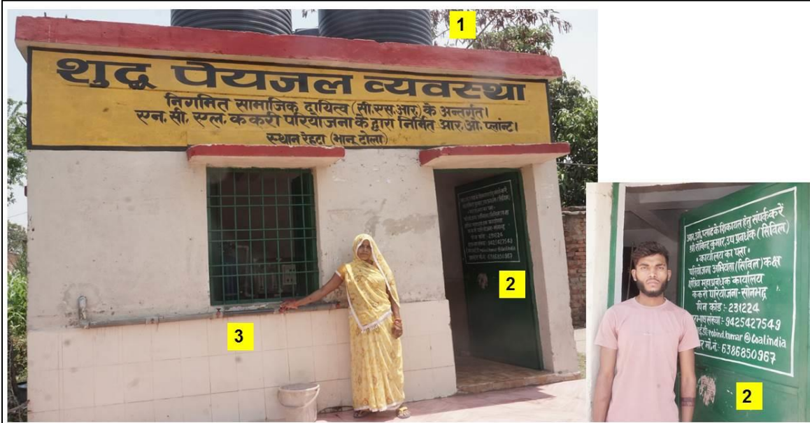
1. Overhead Tank. 2. Contact No. for Complaint & Operator Mobile No. 3. Outlet of Purified Water
