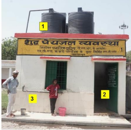
1. Overhead Tank. 2. Contact No. for Complaint & Operator Mobile No. 3. Outlet of Purified Water
