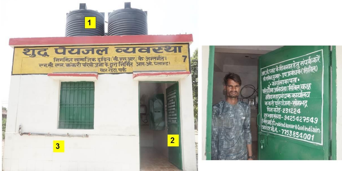
1. Overhead Tank. 2. Contact No. for Complaint & Operator Mobile No. 3. Outlet of Purified Water
